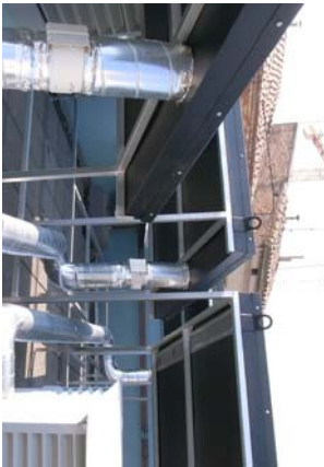
SIMPLE AIR TO AIR SOLAR COLLECTORS MOUNTED ON SOUTH SIDE OF THE EXISTING PITCHED ROOF WILL PROVIDE BACKGROUND HEATING FOR THE RECREATIONAL AREAS AND WARM AIR TO VENTILATE STORAGE AREAS WHERE EQUIPMENT MAY BE DAMP
