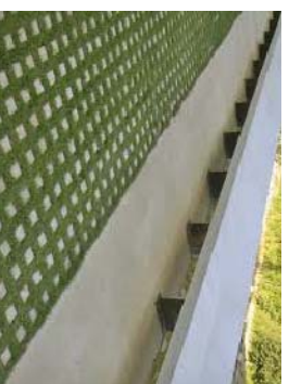
GRASS CONCRETE PAVING IN PARKING AREAS
